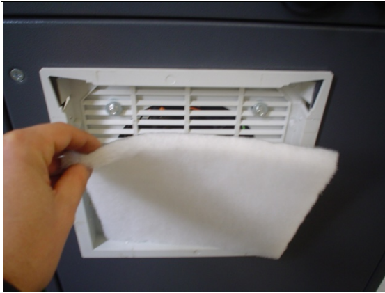
Figure 67:Checking and replacing the dust filter 检查和更换滤尘器
