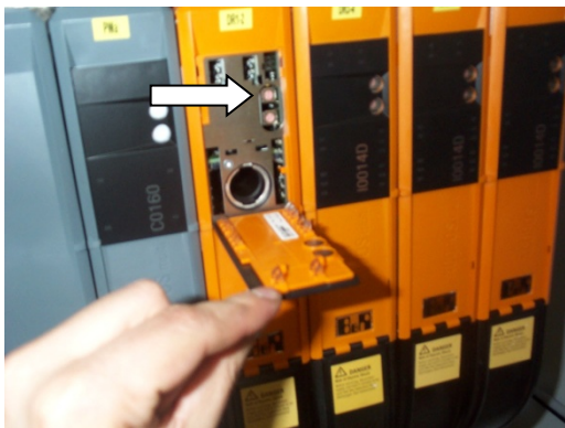
Figure 90: Replacing a drive 更换驱动器
