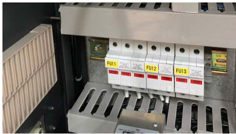
Figure78:Replacing fuses 更换熔断器
