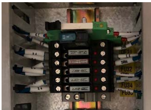
Figure79:Replacing fuses 更换熔断器
