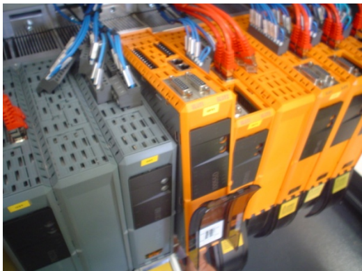
Figure 87:Replacing a drive 更换驱动器
